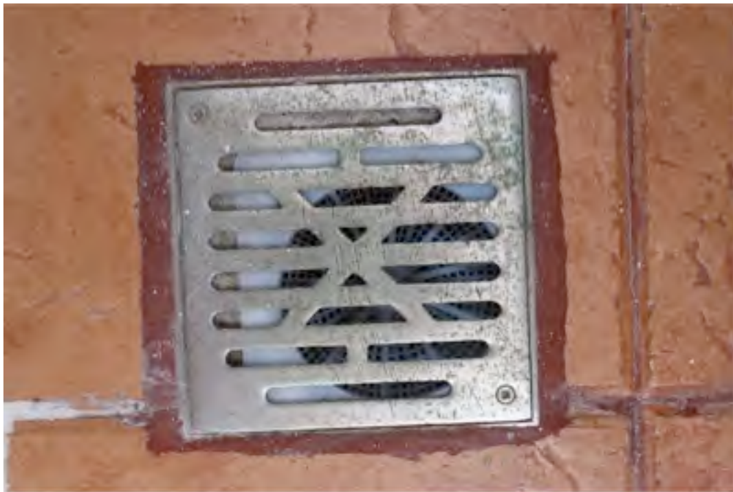
Figure 1 – A typical modern standard grating. Note the smaller plastic mesh underneath to avoid the passage of scorpions.
