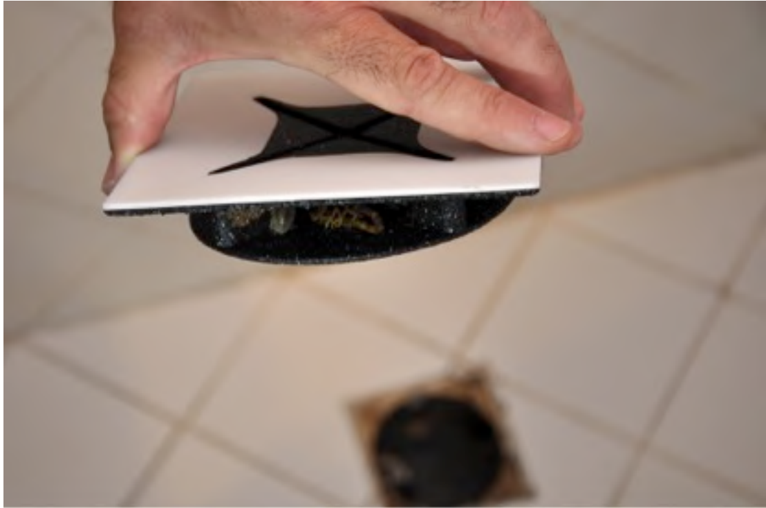
Figure 6 – Taking away the degraded grating.
